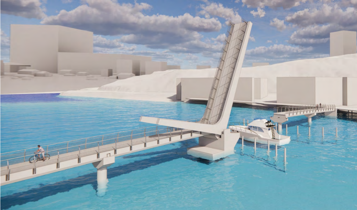
Figure 4-5: View of the bridge from the city side in open configuration
