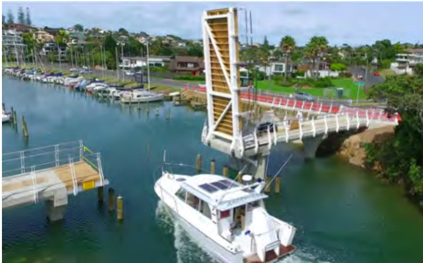
Figure 3-3: Bascule bridge example - Wairau Stream Bridge
