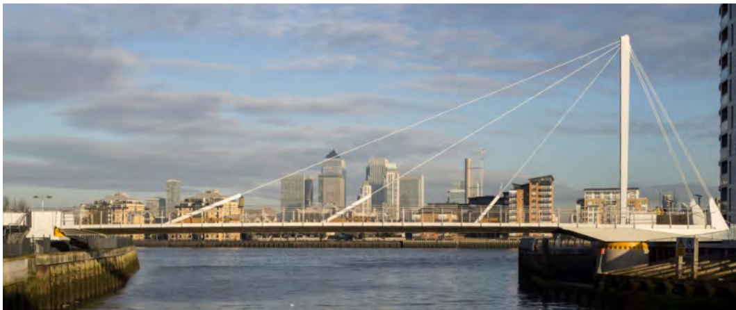
Figure 3-4: Swing bridge example - Deptford Creek Bridge
