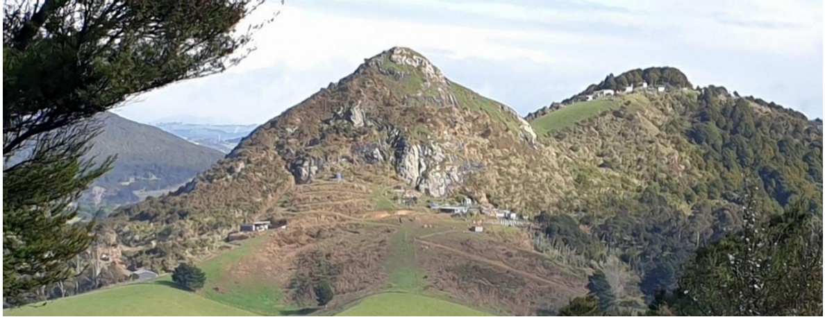
Photograph Appendix C.10: Volcanic rocks exposed on a steep hillslope posing possible rock fall issues.
