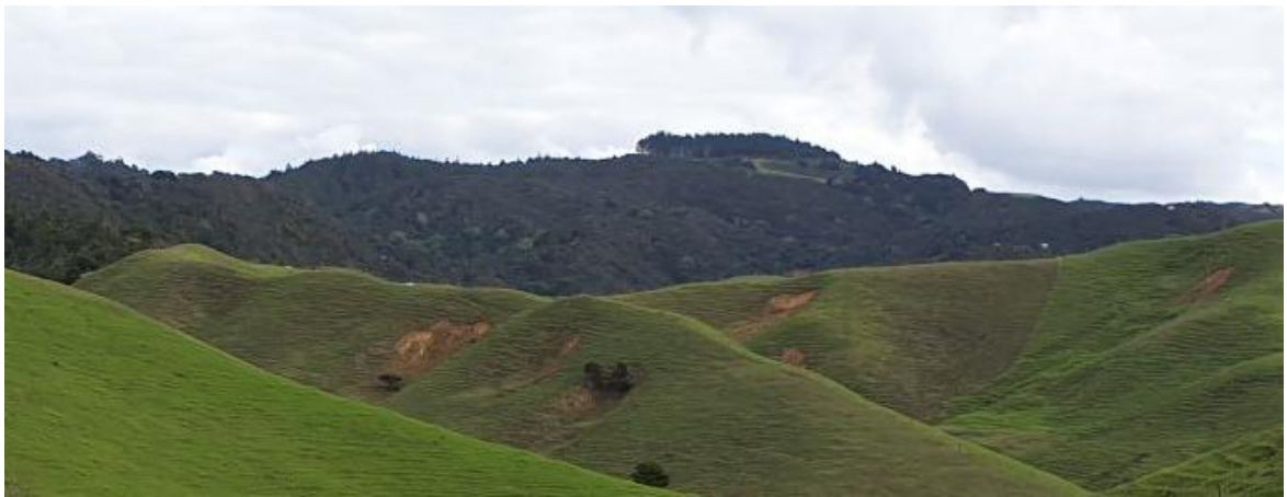
Photograph Appendix C.2: Multiple shallow landslides scarps over the hillslopes.
