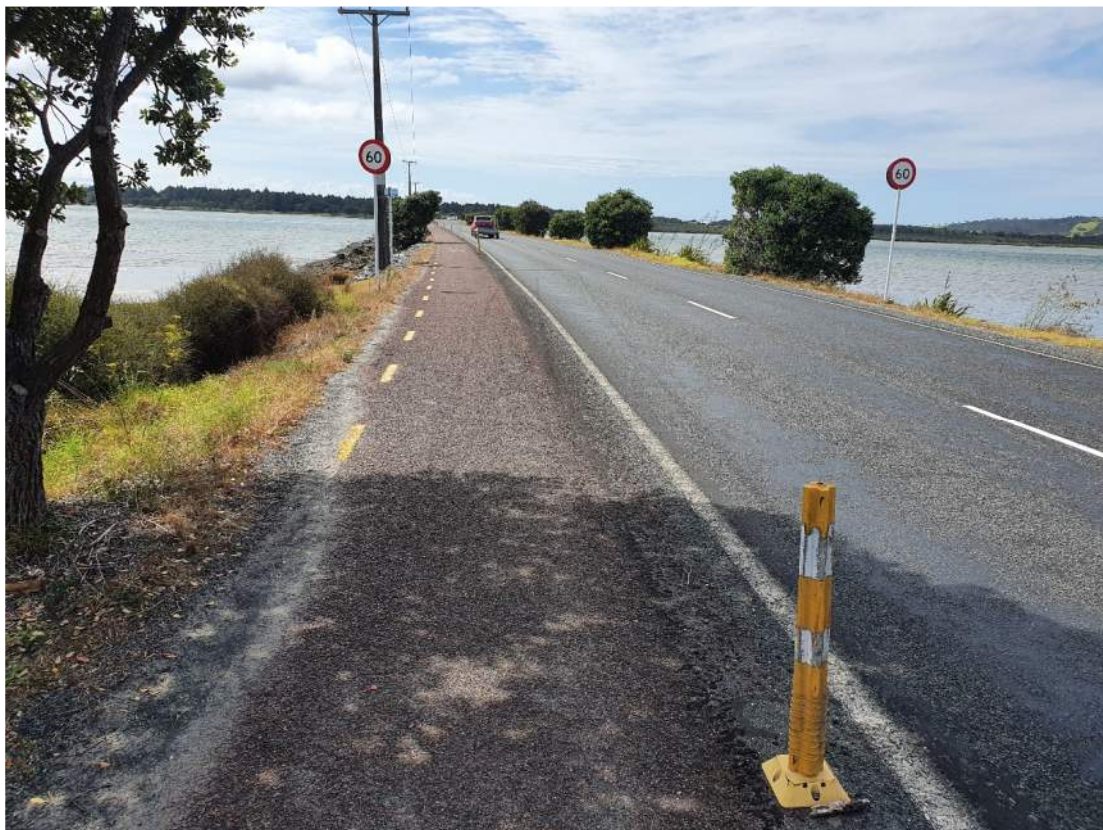
Figure 23: Safe hit posts separate the cycleway from traffic lanes, Broadlands Dr, Omaha
