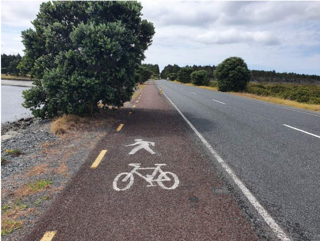
Figure 22: Pavement markings and coloured surfacing delineate the cycleway, Broadlands Dr, Omaha
