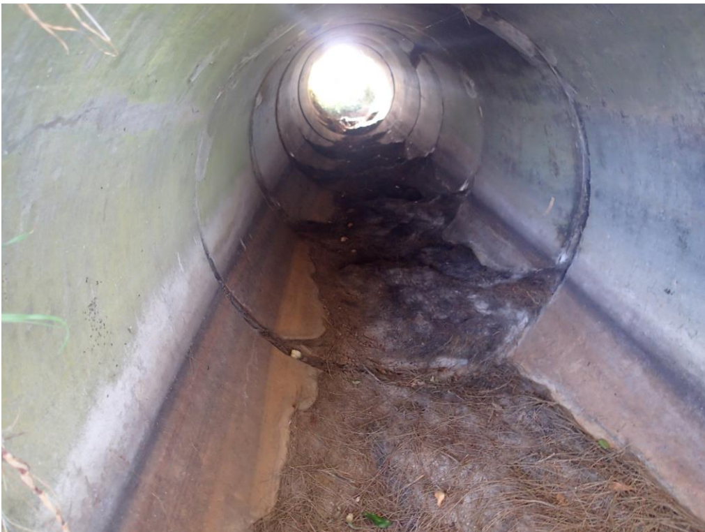
Photo 4. Culvert with natural substrate in base
