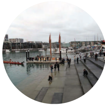
Concrete Terrace Steps
