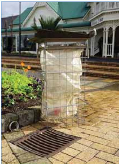
Figure 28 Enviropod, used to filter rubbish coming through stormwater grates, prior to installation
