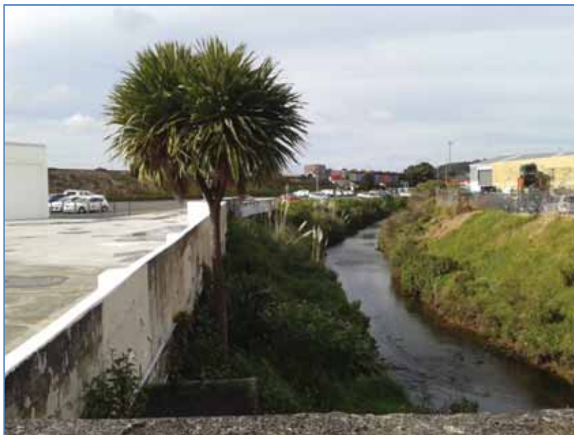
Figure 1 Carpark encroaching on riparian zone, Waiarohia Stream
