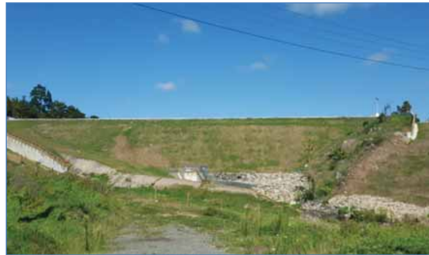
Figure 103 Hopua te Nihotetea Dam viewed from Raumanga Valley Rd
