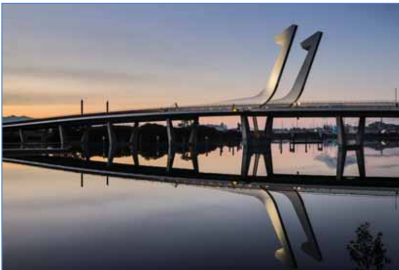
Figure 35 Te Matau a Pohe Bridge
