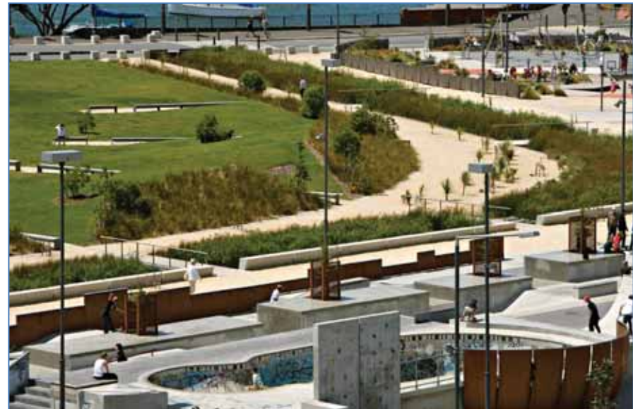
Figure 27 Waitangi Park, Wellington, has a number of small wetlands to filter stormwater prior to entering the harbour
