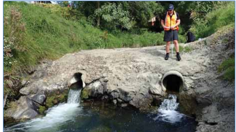
Figure 26 Fish passage barrier on the lower Waiarohia Stream prior to removal in 2015
