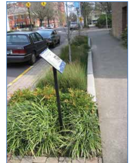
Figure 43 Series of stormwater planters, Portland, Oregon
