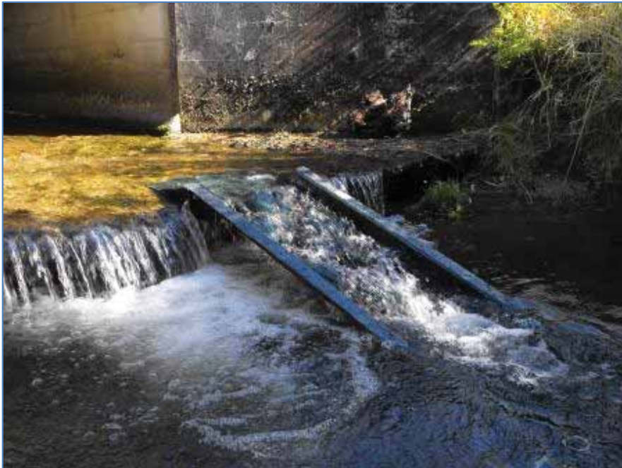
Figure 30 Example of a type of fish ladder, catering to weaker swimmers such as inanga.
