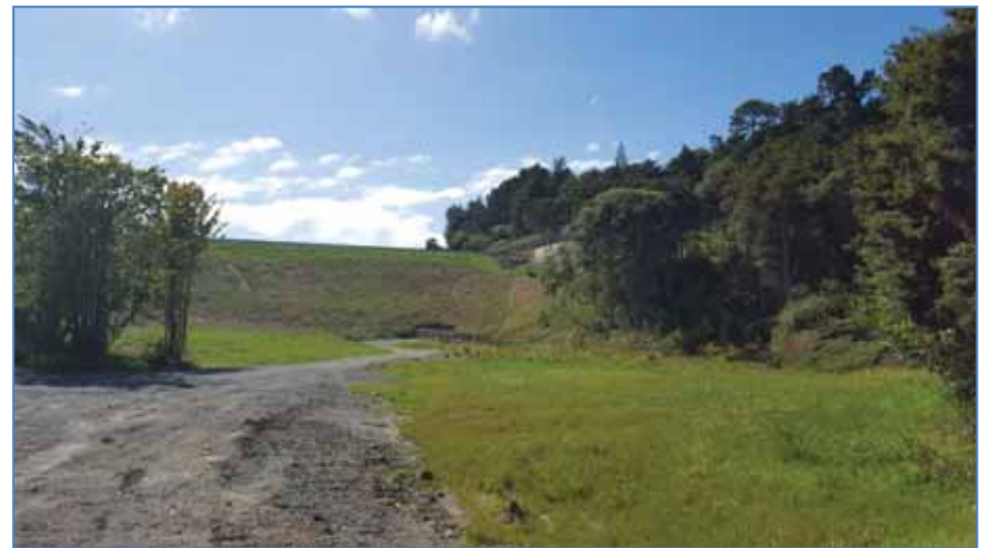
Figure 111 The retention zone at the base of the Hopua te Nihotetea Dam
