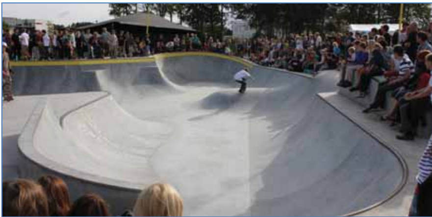
Figure 44 Stormwater retention ponds double as a skatepark, Roskilde, Denmark
