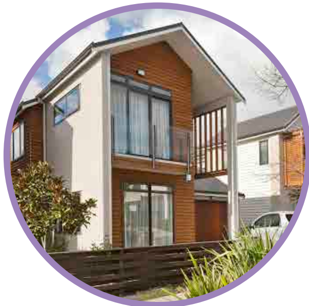
Guideline 2 Hobsonville, Auckland. Eaves are a simple and effective way of protecting wall and roof junctions.
