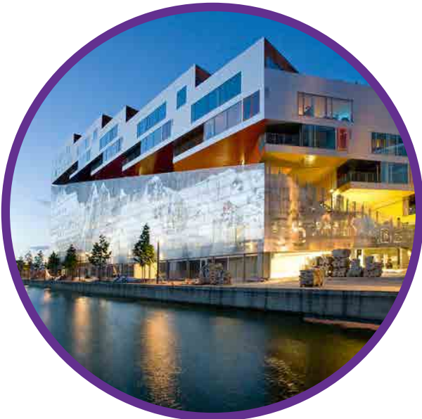
Guideline 11 Mountain Dwellings Ørestad, Copenhagen. This development uses façade detailing to screen above-ground carparking.
