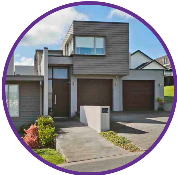
Guideline 8 This double garage does not dominate the house as it is broken up into two and is designed as a part of the façade.
