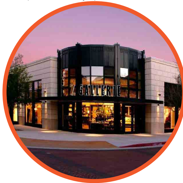
Guideline 5 The building design uses colour, materiality and massing to highlight the building corner and the main entrance.
