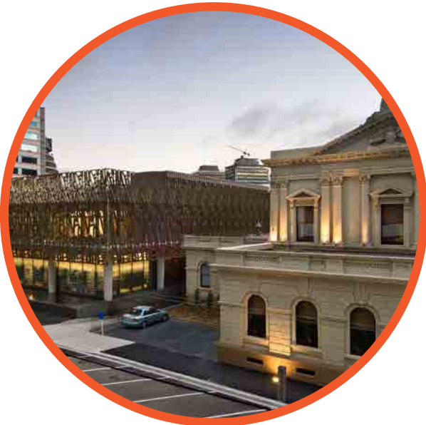
Guideline 1 The Supreme Court, Wellington. The modern extension of the building appears different but maintains the same roof and floor heights.
