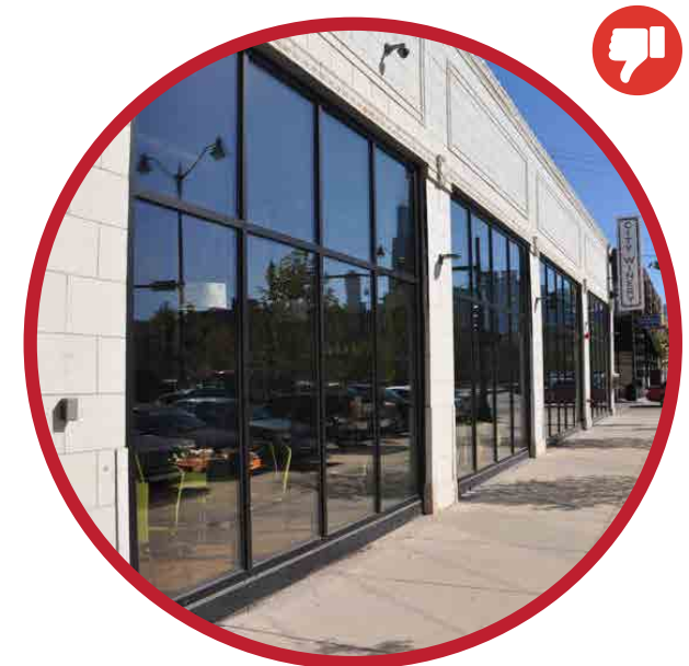
Guideline 3 Tinted windows can disrupt active frontages as they disrupt views which create a presence of people and to street vibrancy.
