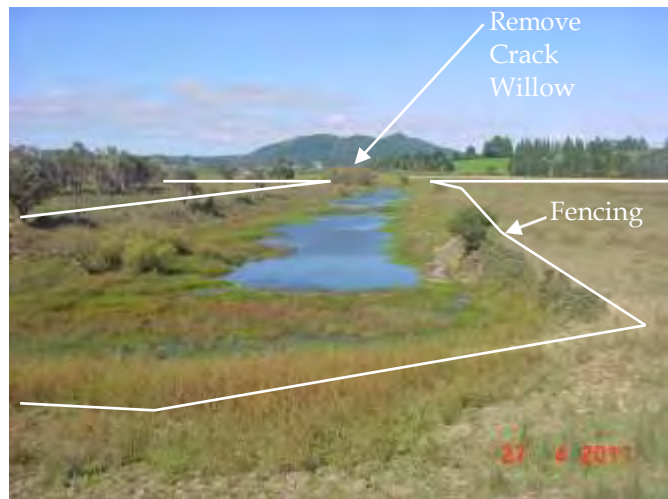
Photo 45: Site 12 - Cut-off Channel Looking Downstream
