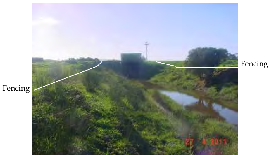
Photo 6: Site 2- Man-made Pumping Channel Looking Upstream
