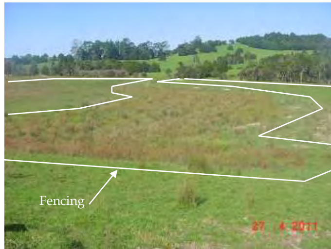
Photo 31: Site 8 - Cut-off Channel Looking Downstream
