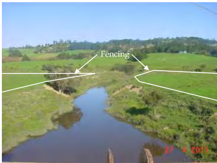
Photo 5: Site 2 - Man-made Pumping Channel Looking Downstream
