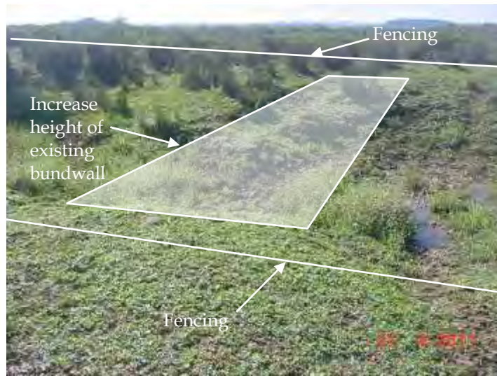
Photo 56: Site 14 - Cut-off Channel Showing Possible Location of Bundwall
