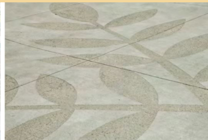
Concrete Patterns contribute to the city's identity: California, USA
